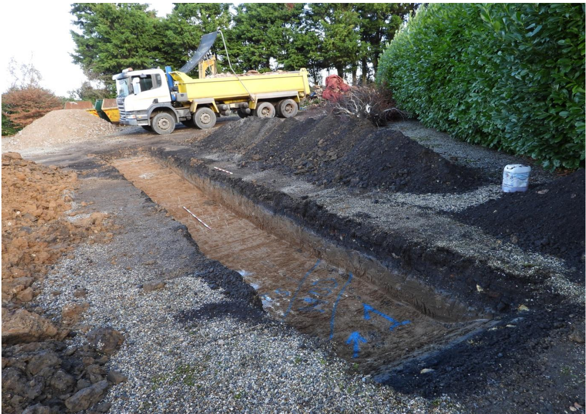
Plate 2: Looking north at trench 1; 2metres scale.
